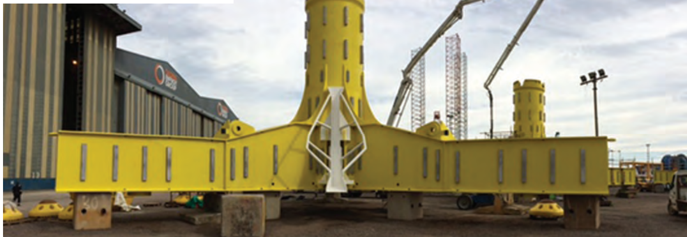
MeyGen turbine foundation complete with anodes for cathodic protection subsea
