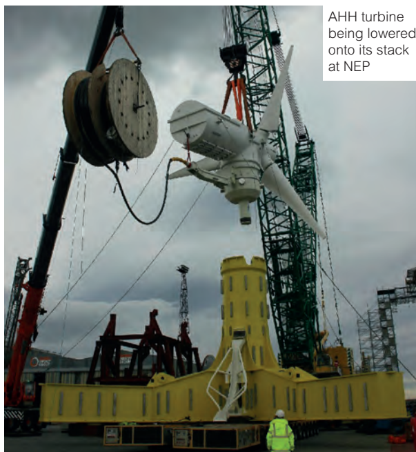
AHH turbine stacked in preparation for deployment at NEP
